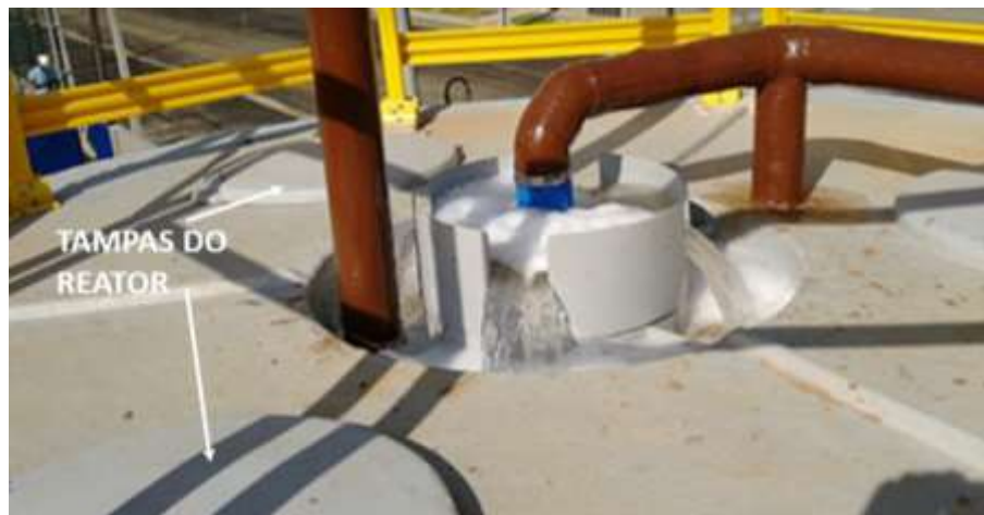
Figura 5: Tampas do Reator MBBR
